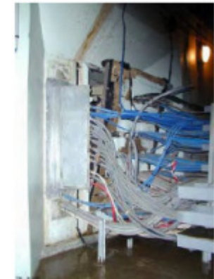
Failure of Cable opening
